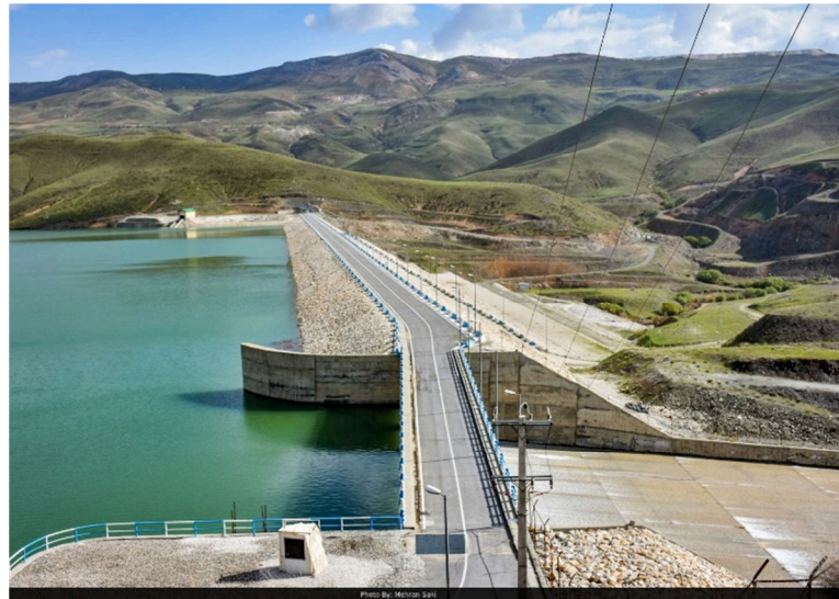
Figure 2. Kamal-Saleh earth dam under overflow condition
