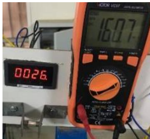
Figure13. Multimeter and power of 10 W.
